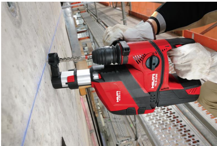
Figure 6: on tool dust extraction (Source: Hilti Australia)
